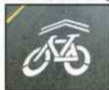
Shared Lane Marking
